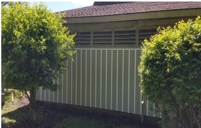
New paneling on the exterior gets attached. It will not be the color depicted in this picture. It will be painted along with the existing trim.
