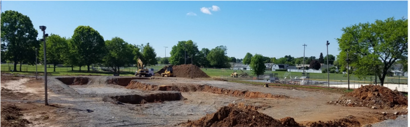
Old vessel is gone and the new form begins to take preliminary shape!
